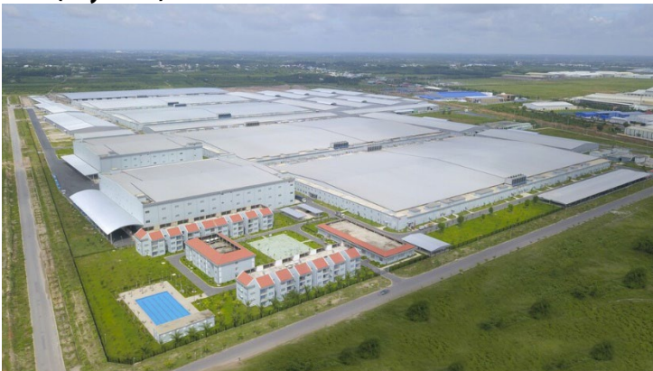
Figure 15: Brotex factory complex in Phuoc Dong Industrial Park (Tay Ninh)
